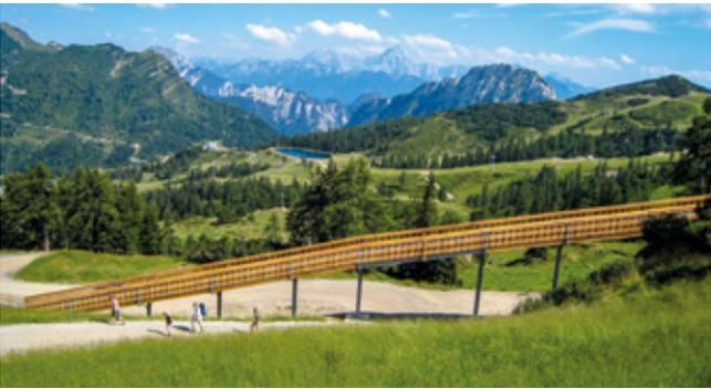
**BRIDGES, TUNNELS AND UNDERPASSES:** They not only serve to optimally adjust the track to the terrain, or to pass over or underneath footpaths or streets, they form an important part of the Mountain Coaster setup.
